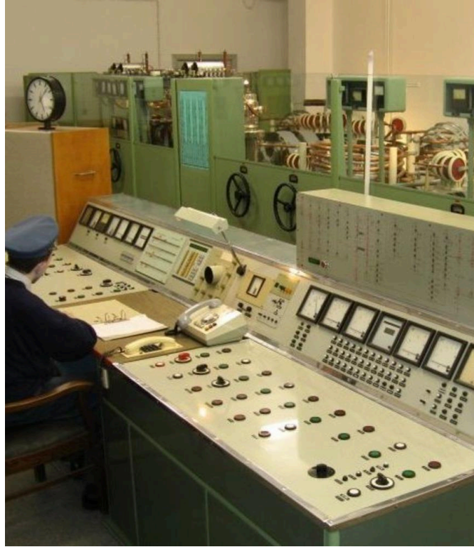
The operator. The console of a broadcast transmitter. Funkerberg Radio Technology Museum.
